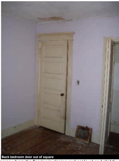
There are areas where the flooring is sloping and not level and slightly uneven indicating some settlement has occurred. The floors are not level and the windows and door frames may not be plumb. see the Foundation section of this report for more information.
