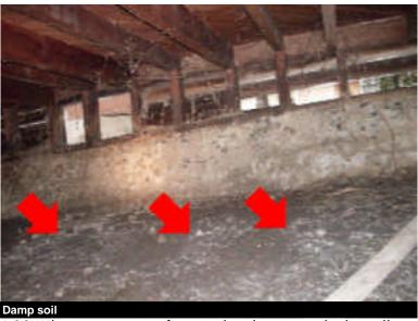
**Not Acceptable**, there are areas of excessive dampness in the soil under the building. This may cause the building to feel damp and create the growth of mold and/or mildew. It is typically advised to have this examined by specialists to have the source of the moisture detected and any needed corrections performed plus any growth properly abated.
