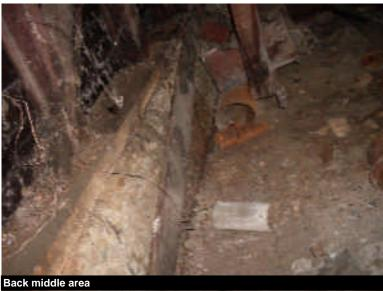
Needs Attention, The structure is not bolted to the foundation. Ideally foundation anchor bolts would be added to attach the wood frame of the building to the foundation to prevent movement in case of seismic activity.
