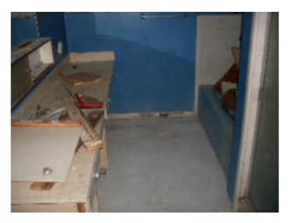
The toilet has been removed, and there is debris from partial demolition of the sink and cabinets and the tub is filled with debris.
