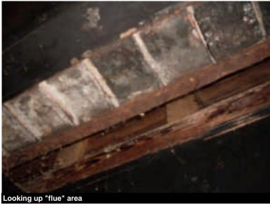
**Not Acceptable:** , the flue vent pipe has been removed and this can not be used and would require extensive work to modify and install a new gas appliance system.
