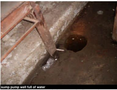
**Not Acceptable**, there is water percolating up at the floor and concrete wall and water is ponding on the floor.
