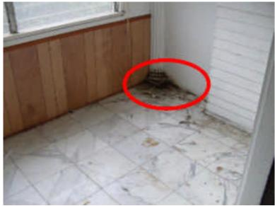
Needs Attention, there are areas of moisture stains, on the wall and bottom corner (the window with the awning is just outside of this area)
