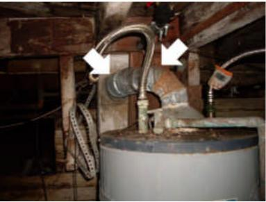
Needs Attention, the vent line from the water heater has a negative fall and the gases will not vent properly. This is a safety hazard and needs to be repaired.
