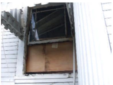
The awning over the right window near the enclosed porch appears to have re directed the water run off onto the column area, the wood is damaged and there are moisture stains in the corner inside
