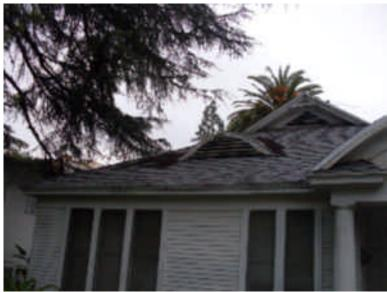
It was reported that the roof is about ten years old. There are obvious signs of neglect and excessive vegetation on the roof. There are no gutters and poor drainage control.
